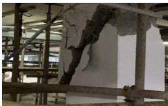
柱受剪裂缝
